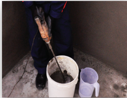
Mix Ezi PLASTER BASE with clean water as per recommended ratio.
