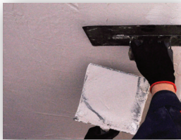
Level, compact and smoothen the plastering mortar with steel trowel.
