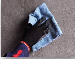
Ensure the substrate is dry, flat and free of contaminants.
