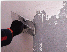
Spread at 2-4 mm per layer each time.
